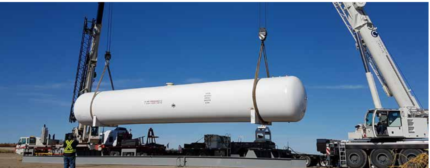
LANDING A 45,000 GALLON STORAGE TANK
