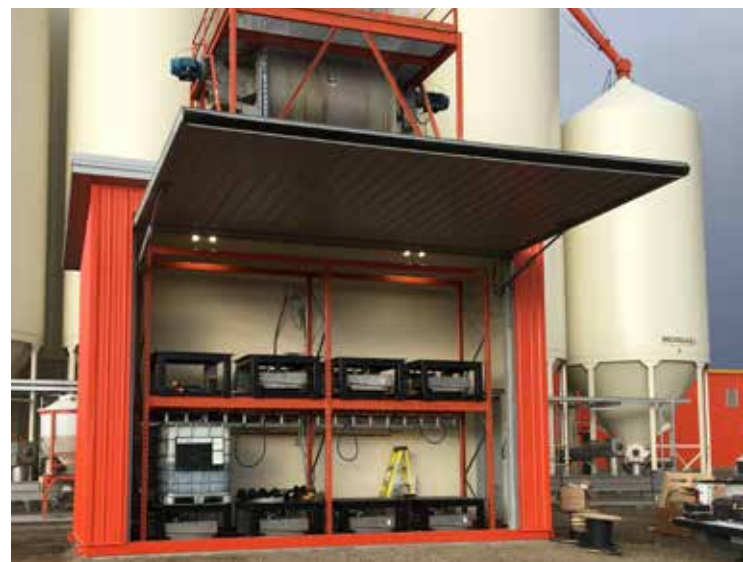
8 SKID SET-UP IN A HEATED SHED
